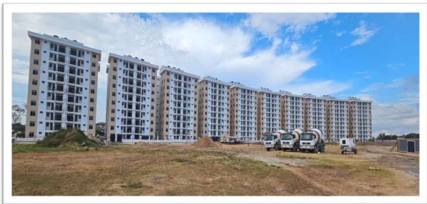
Mradi wa Samia Housing Scheme, Kawe Dar es Salaam
